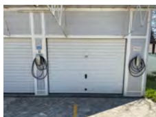
E Charging Station Free charging for guests! Hausgäste laden gratis!
